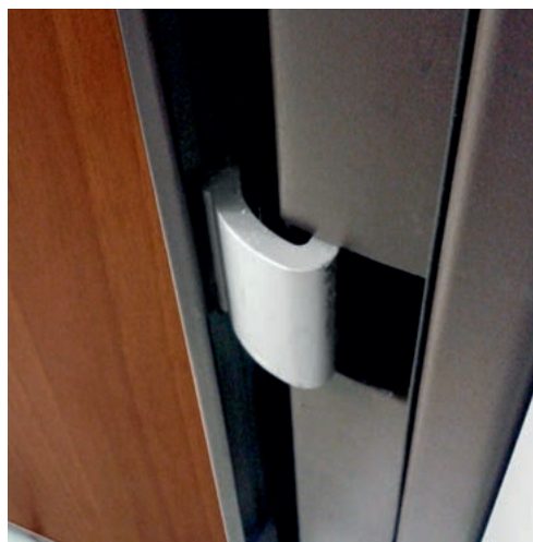
CERNIERA A SCOMPARSA CONCEALED HINGE
