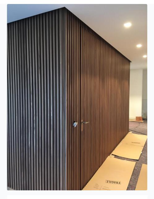
Infinity System is a wall cladding boiserie made of flush facing panels and swing doors: when doors are closed the entire system is a continuous wooden cladding without any visible fitting.
