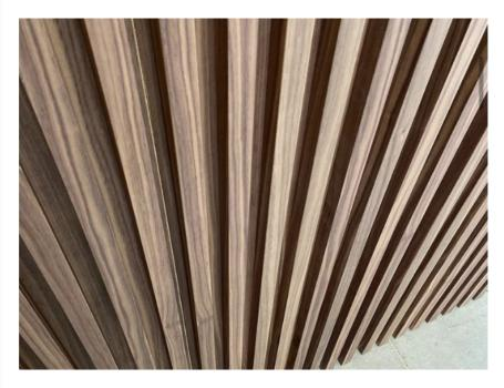
The new wall cladding solution proposed by Ghizzi&Benatti is called T25, as it is made up of vertical slats measuring 25x25 mm.
